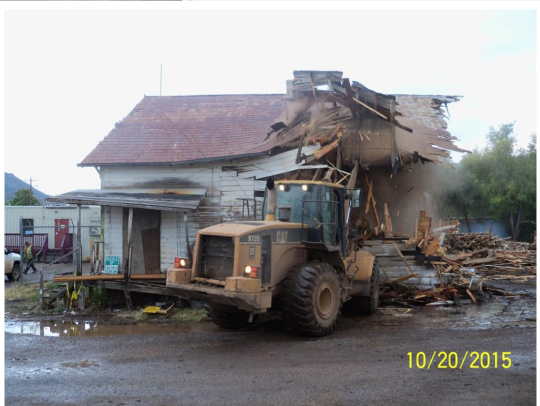
During demolish of building by Tribal Public Works Department.
